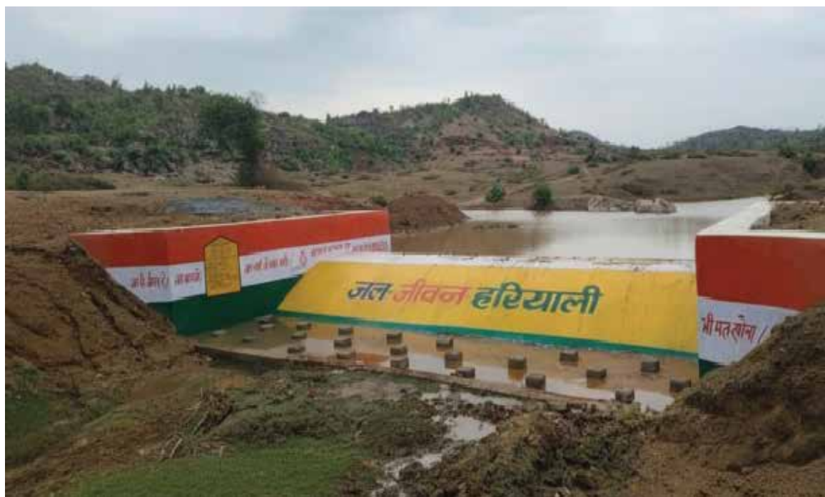
Construction of Checkdam in Gaya ji District of South Bihar
